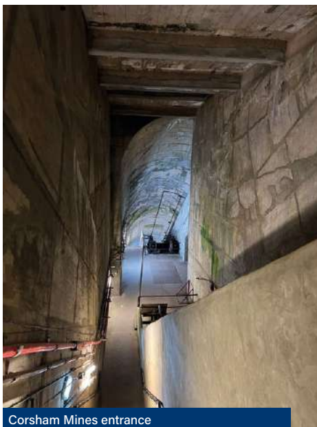
Corsham Mines entrance
