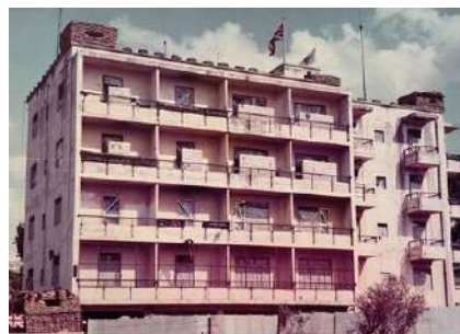
La Regie before rocket screens. Author's room can be seen on top floor – without the outside balcony wall!
